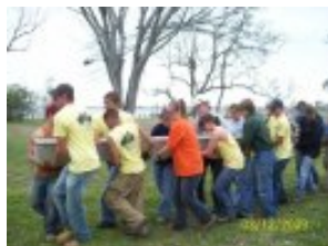
CSC students work together to haul a section of cinder-block foundation from a residential lot
