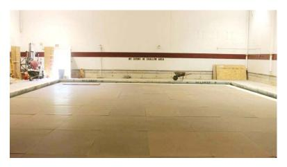
The pool at Armstrong Gymnasium full of foam prior to the concrete floor of the new strength and conditioning center being poured.
