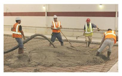
Crews shown May 30 pouring concrete over the foam filling the former Armstrong pool. This area will become the floor for a new strength and conditioning center.
