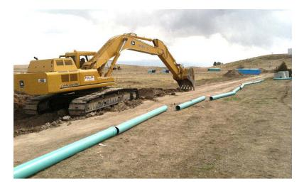
Equipment digging trenches for water and sewer to Eagle Ridge housing and the Coffee Agriculture Pavilion.
